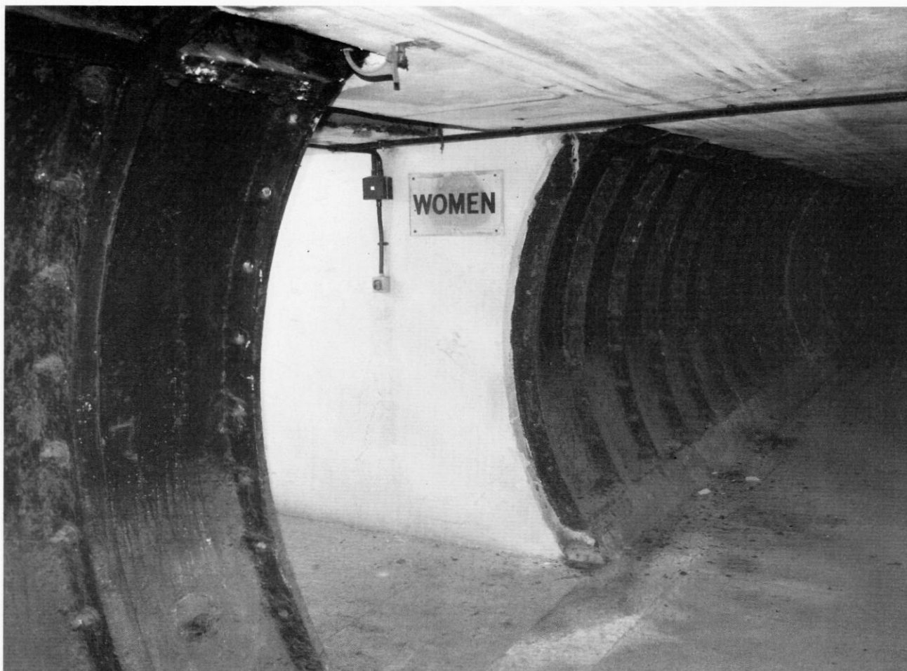
Lower level, entrance to women's toilets
